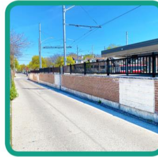
Separation wall with brick portions
