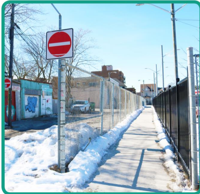
Existing Condition of Walkway
