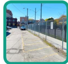
Fence separating walkway
