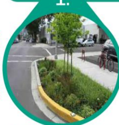
Traffic separation planter
